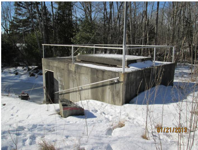
View of Turbine Building (Site Building). View is to the southwest.
