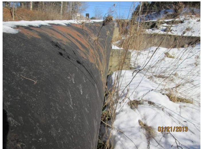
Black mastic/sealant applied to exterior of penstock piping (Samples MAS-02A through MAS-02C)
