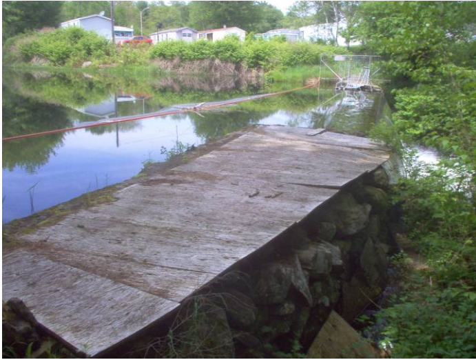
View of the Kelly Dam. View is to the northeast.
