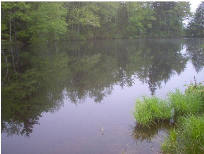
View of Lower Mason Pond in the Goose River behind Kelly Dam. View is to the north.
