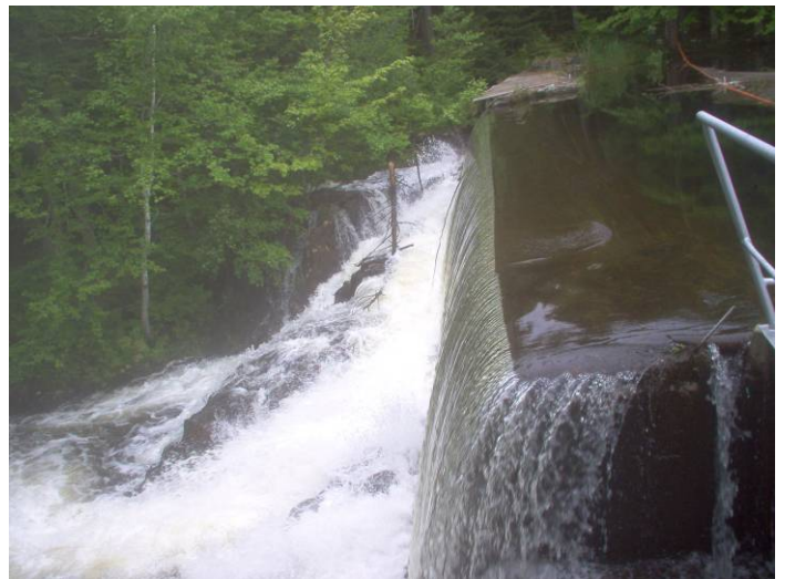
View of the outfall of Goose River over Kelly Dam. View is to the west.
