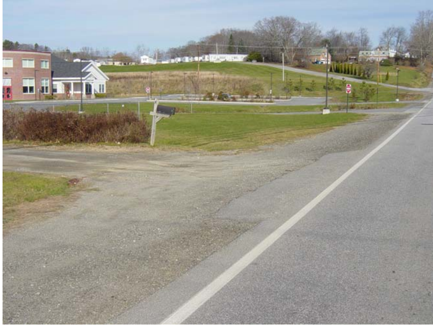
Figure 6. Sidewalk on Rt. 141 ends at Robbins Rd. instead of at the East Side school or Keene Mobile Home Park
