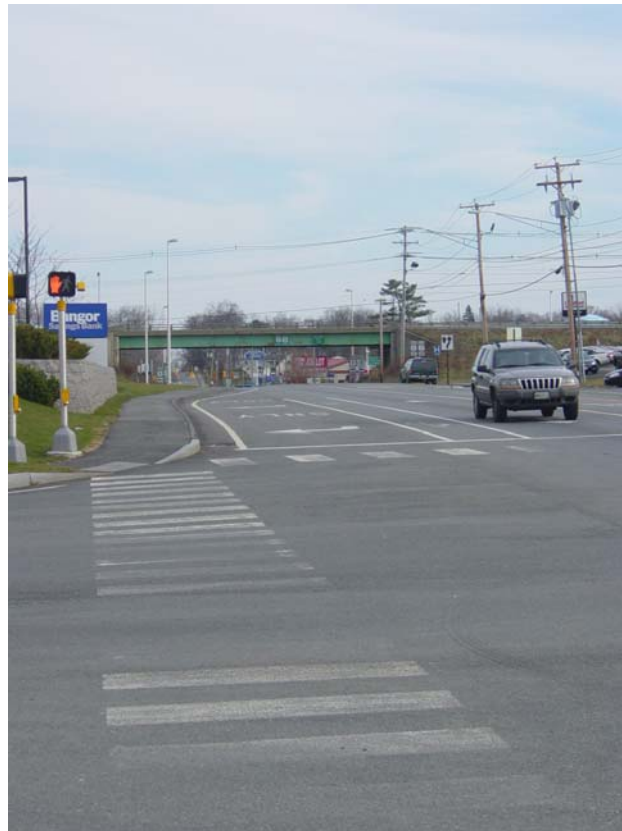
Figure 4. The new Reny's entrance has turn lanes, bike lane, and pedestrian signal
